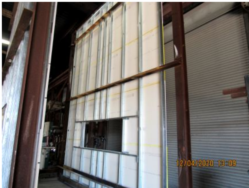
Photo No. 2 Exterior sheathing installed
