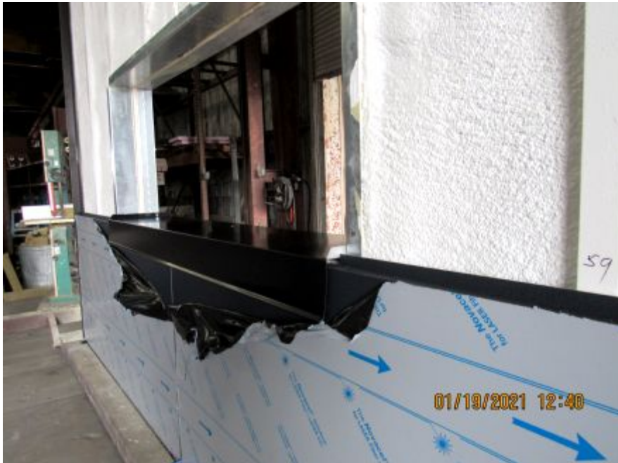
Photo No. 18 Panel assembly
