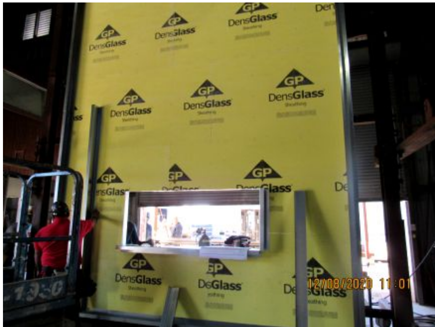
Photo No. 8 Installation of Z-girts
