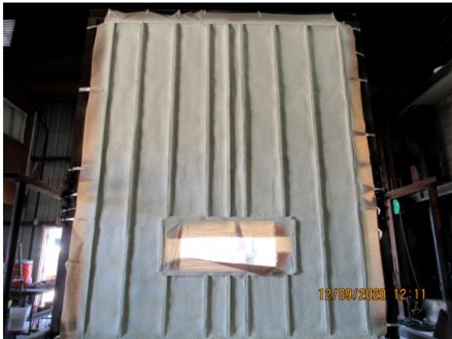
Photo No. 14 Spray foam complete
