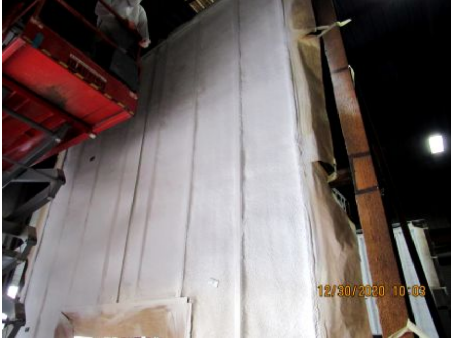
Photo No. 17 Spray complete
