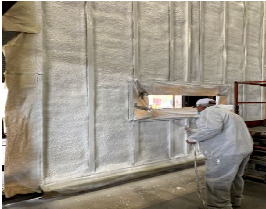
Photo No. 16 Spraying DC315
