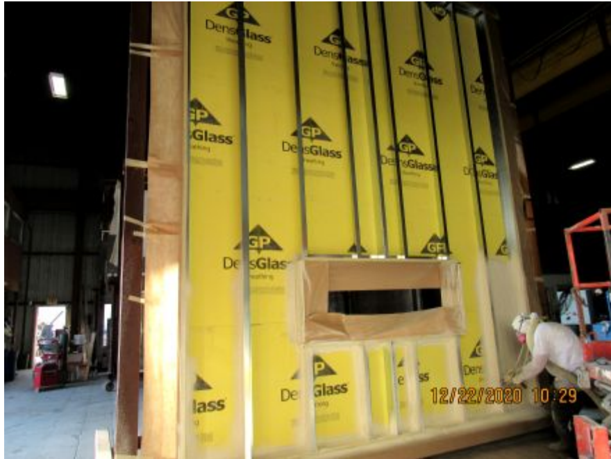
Photo No. 11 Wall pre-foam spray
