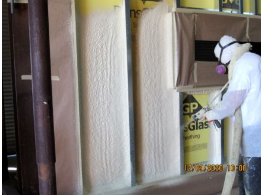
Photo No. 13 Application of spray foam
