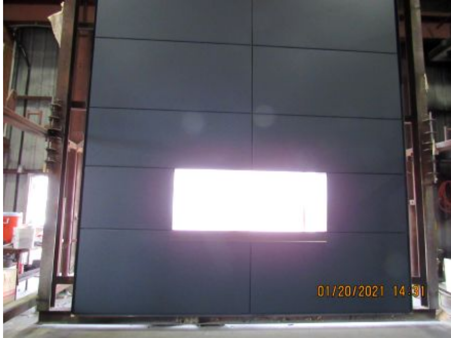
Photo No. 19 Wall assembly complete
