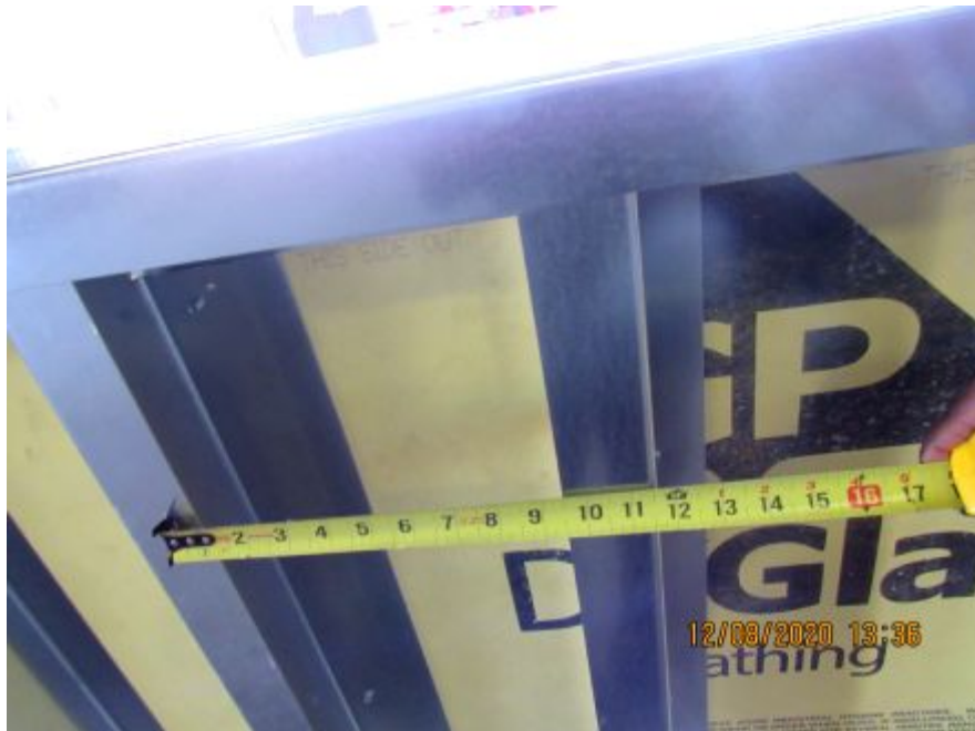
Photo No. 10 Z-girt spacing
